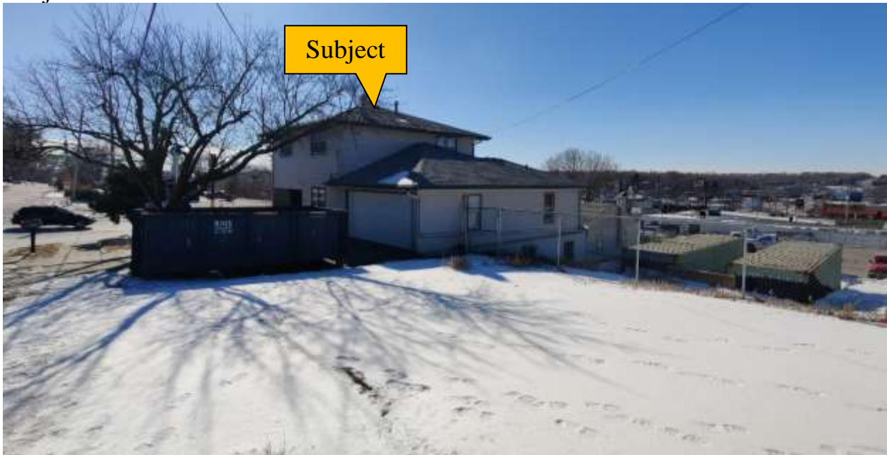
Looking south on North 83rd Street on the north boundary
