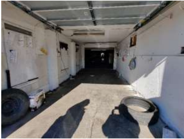
Storage Access Bay 2
